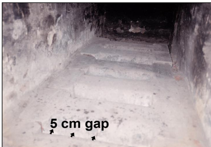
Illustration 37: Interior of the Topf Company furnace, type Auschwitz, with slits in the fireclay grate with a width of merely 1.97 inch.
