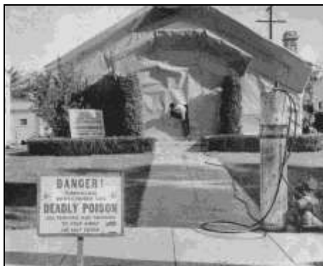
“How to get rid of termites,” Life magazine, 22 December 1947, p. 31. A house in the U.S. wrapped up for disinfestation with hydrogen cyanide piped in from an industrial-size steel bottle.
