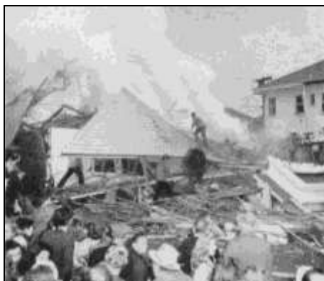
Same scene, a short while later: The concentration of hydrogen cyanide used was too high. One single spark, and the entire house blew up.
