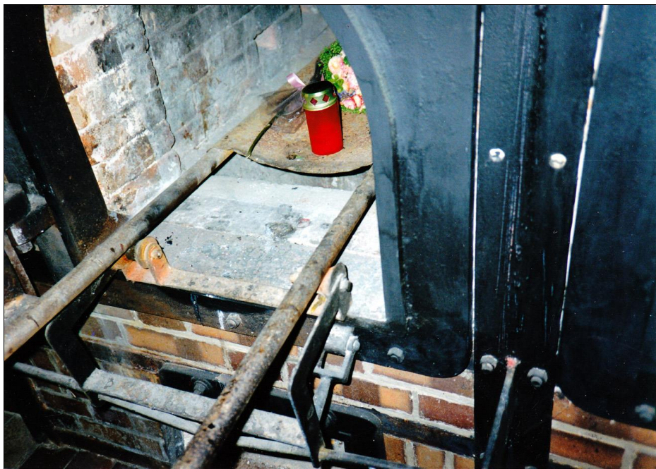
Document 12: Corpse-introduction stretcher in the left muffle of the double-muffle Topf Furnace at CC Mauthausen, resting on a pair of guide rollers. Mattogno/Deana, Part 3, Photo 85, p. 68.
