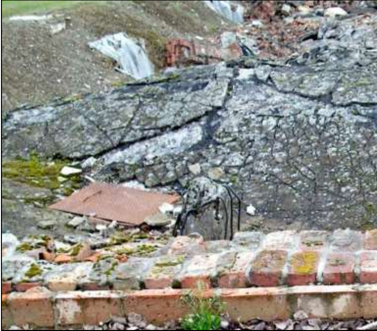
Photo 10: Steel lid of an inspection port on the roof of Morgue #2 of Crematorium II in Birkenau. © C. Mattogno.
