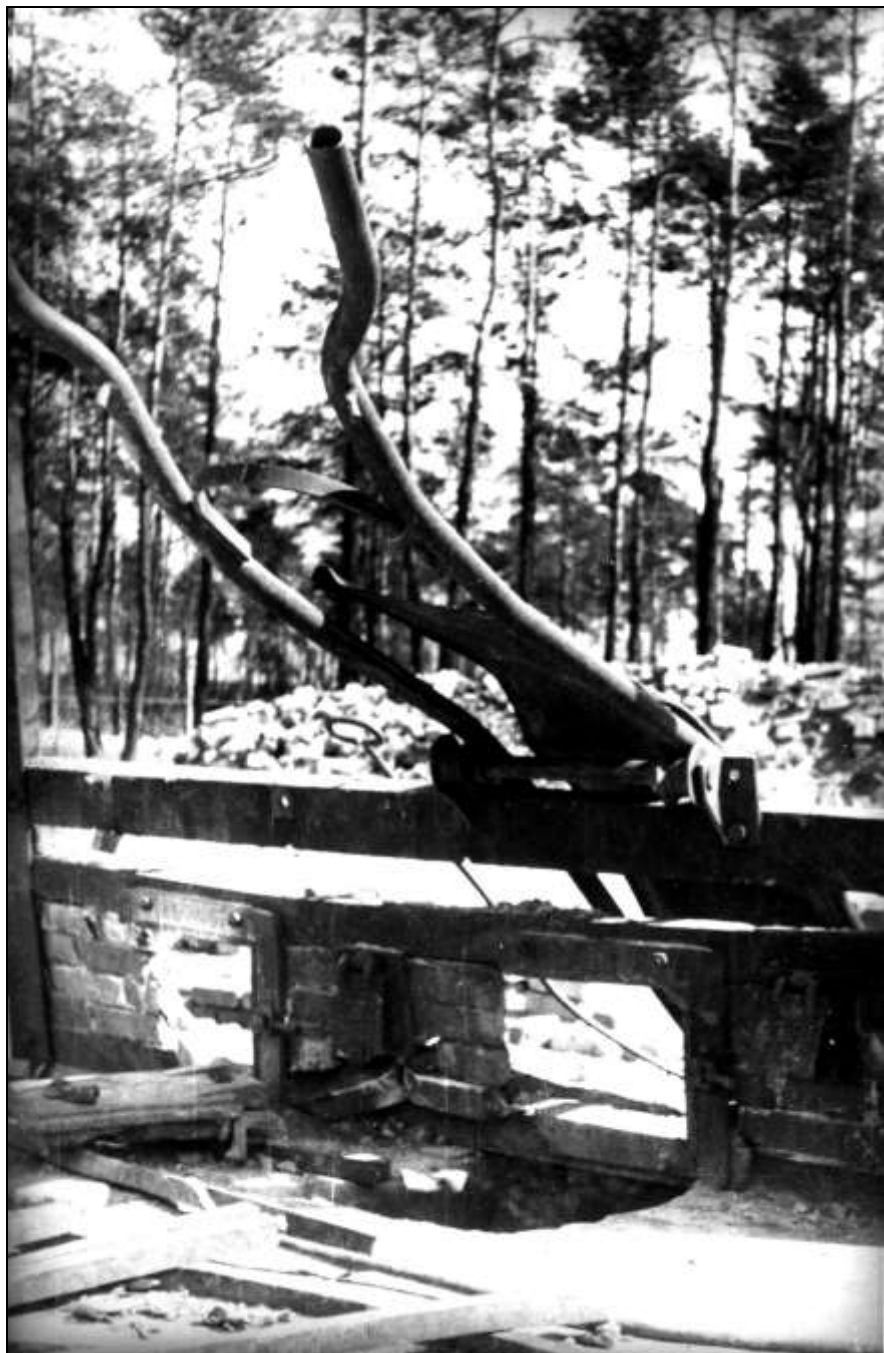
Document 16: Ruins of Crematorium V. Polish photograph of 1945. APMO, Negative No. 859.
