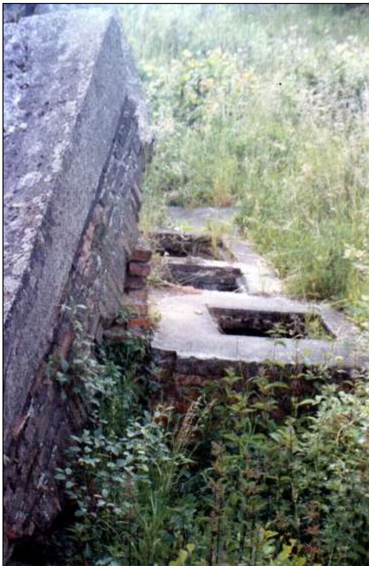
Photo 9: Inspection shafts in the ruins of Crematorium III at Birkenau. © C. Mattogno.
