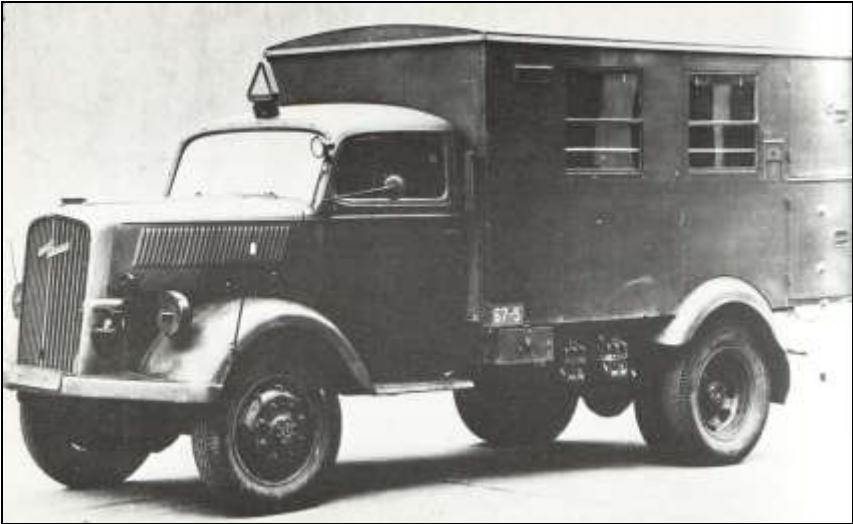
Illustration 26: Opel Blitz, A-Type (=all wheel drive), 3 tons. Together with the S-Type (standard drive), almost 100,000 of this truck were delivered to the Wehrmacht during World War II, some built by Daimler Benz, Borgward, and Klöckner-Deutz under license. It came with a broad range of coachworks. Hence, there was nothing special about this truck at all. Engine: gasoline, 3,600 ccm, 6 cyl., 68 HP. With such an engine, its exhaust gases were lethal. (Picture from Mil-som 1975, p. 174)
