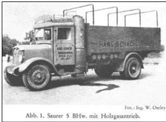
Illustration 3: A German wartime producer gas truck form Saurer (Type 5 BHw, produced until 1935; Berg 2019, p. 465)
