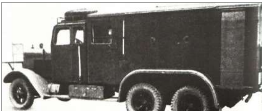
Illustration 24: Sd.-Kfz 92, personnel decontamination vehicle, Henschel 33G1 (picture from Milsom 1975, p. 144).
