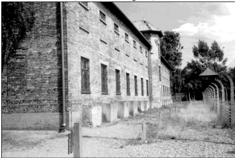
Photo 26: Block 11, outside, wall facing SSW, concrete screens around the window wells of the bunker cells.
