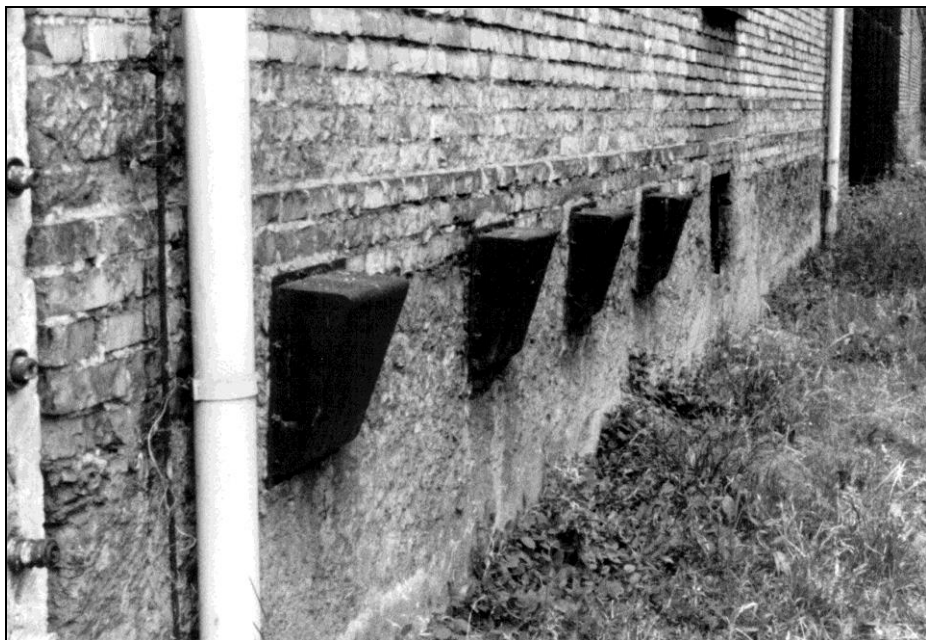
Photo 30: Block 11, outside, wall facing SE, sheet-metal boxes covering the air-supply holes of the 4 stand-up cells of the bunker.
