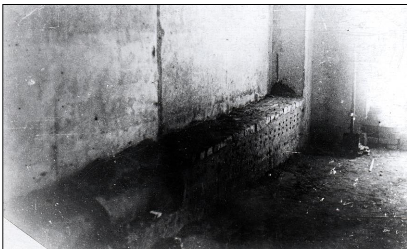
Photo 10: The interior of the disinfestation chamber at Stutthof, west wall: cast-iron connection pipe to the stove located outside the delousing chamber and used to heat the air inside the chamber. Half of it is covered by perforated bricks.
