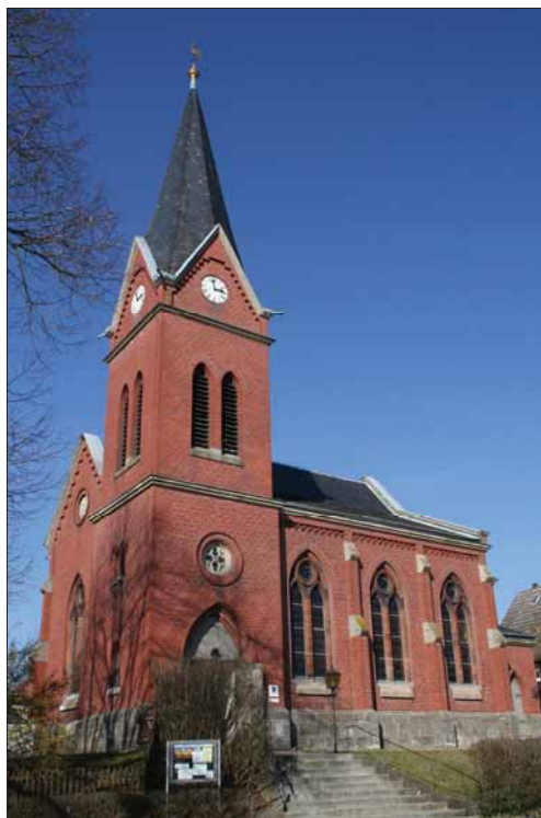
Figure 8: In August 1976, the Protestant church at D-96484 Meeder-Wiesenfeld was fumigated with Zyklon B. Subsequently, blue-colored stains appeared all over the plaster (see Figure 9).
